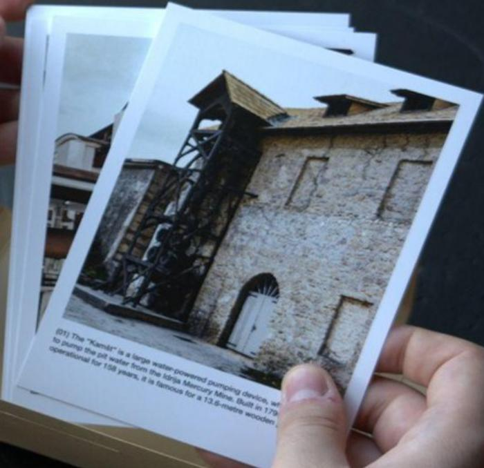
(01) The "Kendi" is a large water-powered pumping device, set to pump the pit water from the Sirisa Mercury Mine. Built in 1790, operational for 158 years, it is famous for a 12.9-metre wooden
